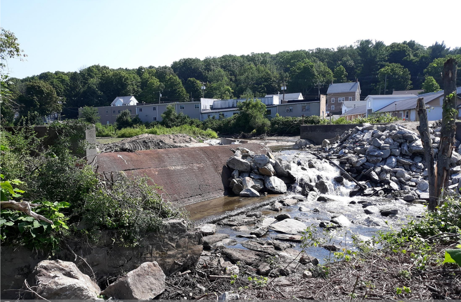
As the impoundment drained, all upstream flow from Steele Brook was directed to a tributary along the east bank of the former impoundment
